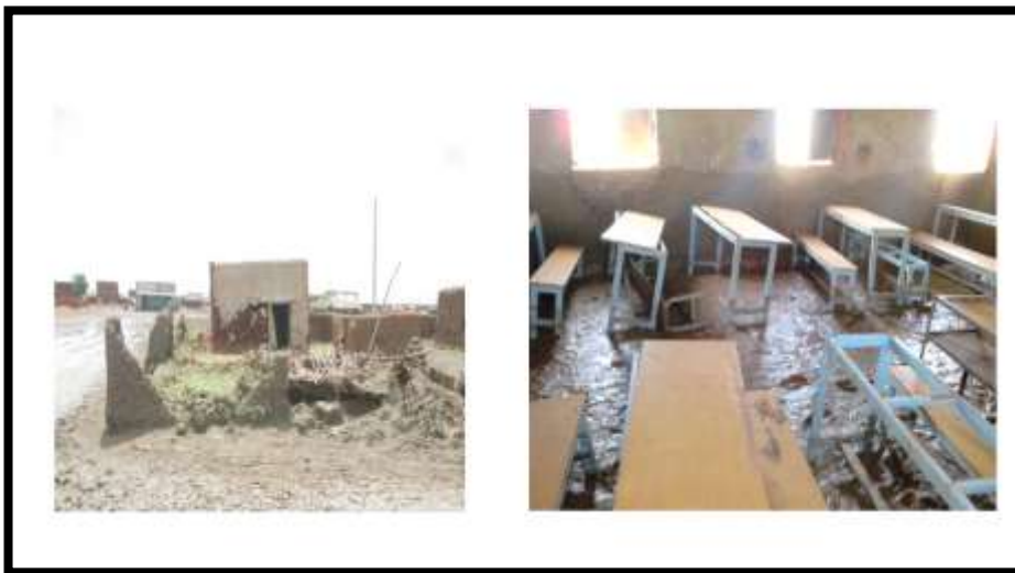
Figure 2: Damaged house, pit latrine & school.
